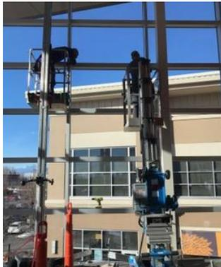
Between January 10 and January 19, our facilities techs Matt James and Rob Stansbury worked with electricians and shade installers to replace lights and install window blinds in CTL's atrium. The new lights are energy-efficient LEDs that shine brightly from the 60' ceilings, giving the area a more welcoming and clean feel. The window blinds have the opposite effect: they block our powerful winter sun in the afternoons, making computer monitors easier to see and easing eye strain.
